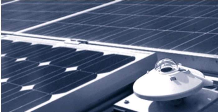
Fig. 3: Tilted pyranometers used for plant performance modelling on a PV plant
