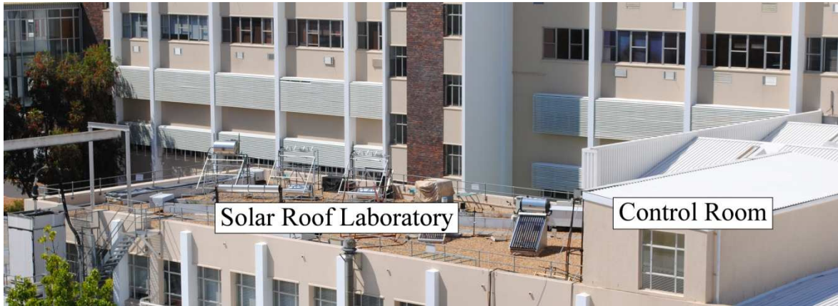
Fig. 1. Overall view of the Solar Roof Laboratory from the North.
