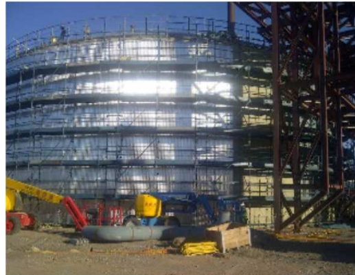
Molten salt storage tanks
