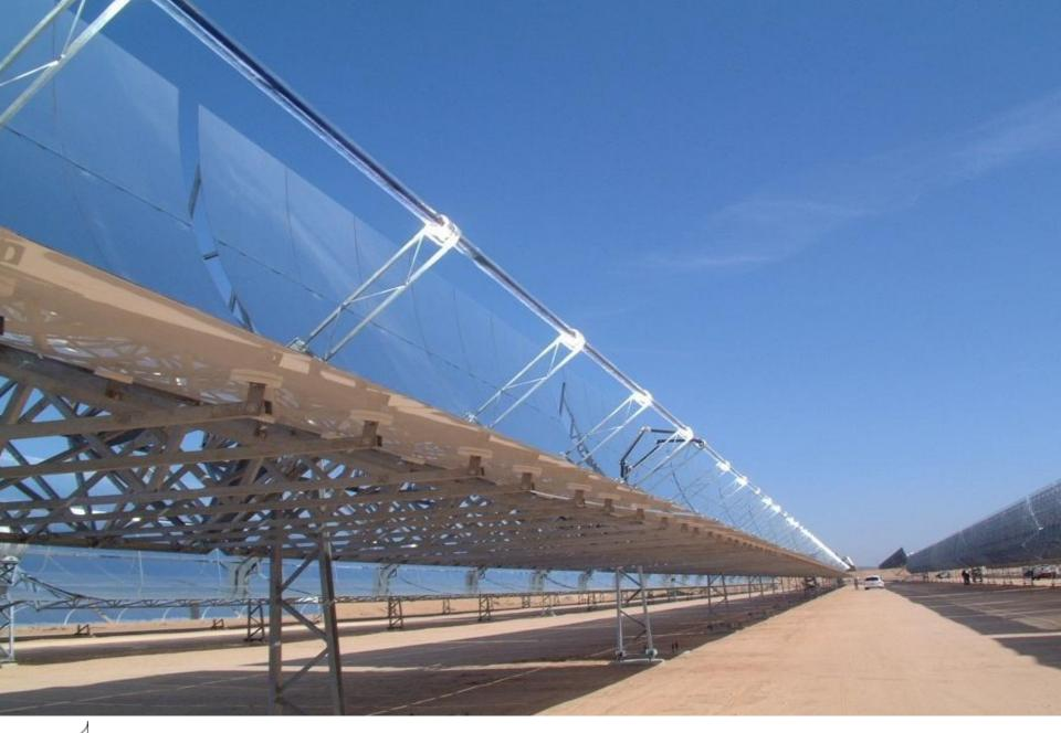
SKAL-ET loop integrated in the SEGS V plant in California
