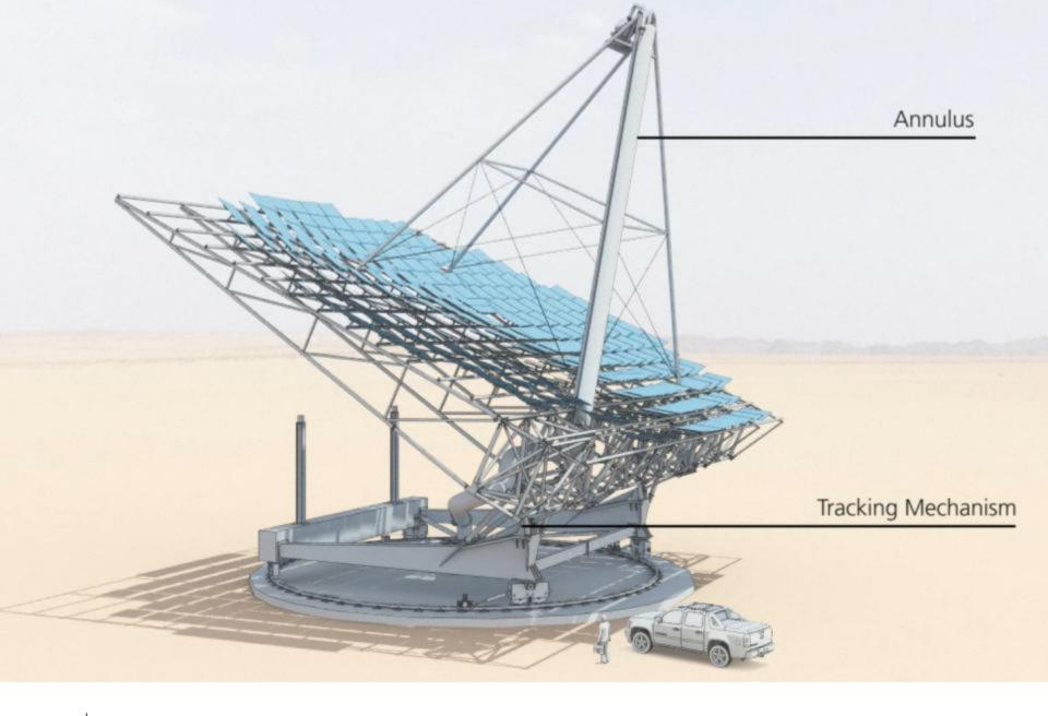
HelioFocus solar concentrator – 500m<sup>2</sup> fresnel dish
