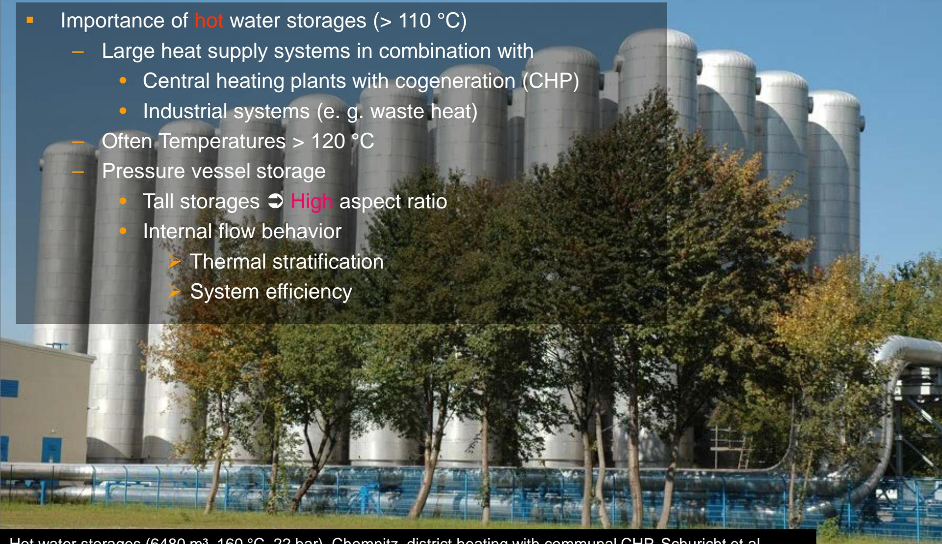
Hot water storages (6480 m<sup>3</sup>, 160 °C, 22 bar), Chemnitz, district heating with communal CHP, Schuricht et al.
