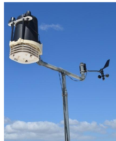
Fig. 2 A Davis weather station system installed on top of the 18m Tower at Stellenbosch University
