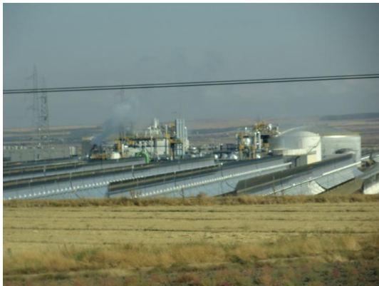
Figure 1: Andasol 2 in Operation
