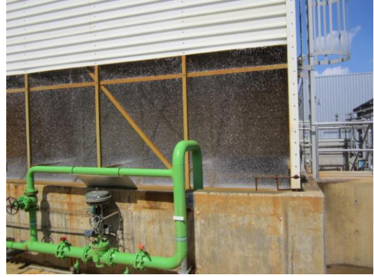
Figure 16: Wet cooling system up close
