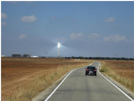
Figure 9: Approaching the plant where the heliostats can be seen the first time
