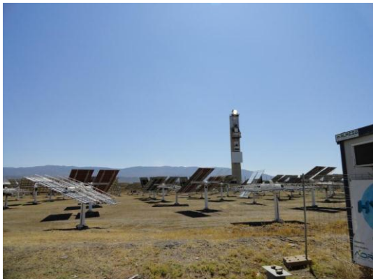
Figure 6: Plataforma Solar (Field 1 of 2)
