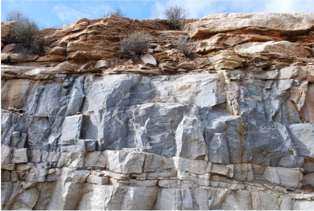
Figure 10: Cutting on the N7, showing strata/layer separation
