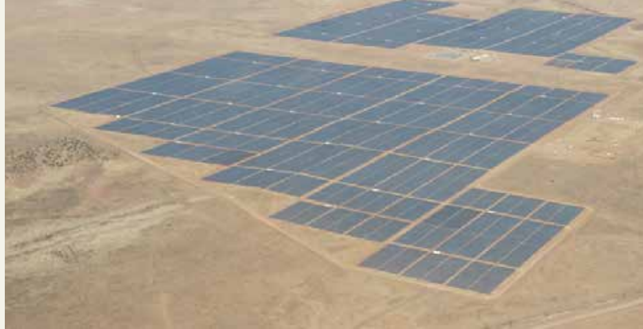
Figure 10: Dreunberg 75MW photovoltaic power plant. Scatec Solar, South Africa (Scatec Solar 2014).
