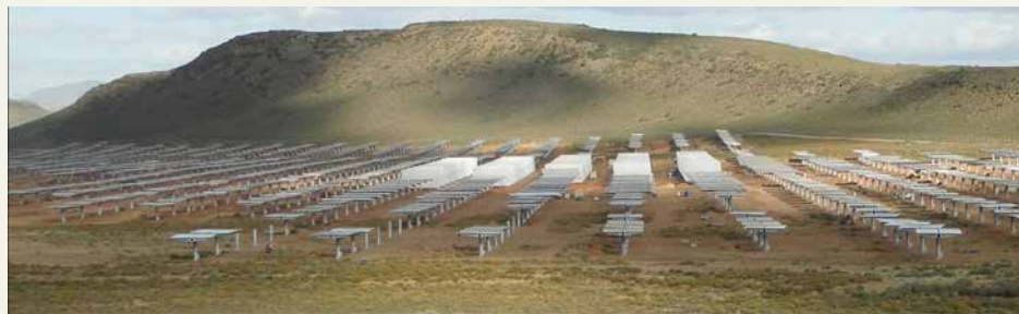
Figure 11: Touwsrivier 44MW concentrated PV facility under construction. Soitec, South Africa (CRSES n.d.).
