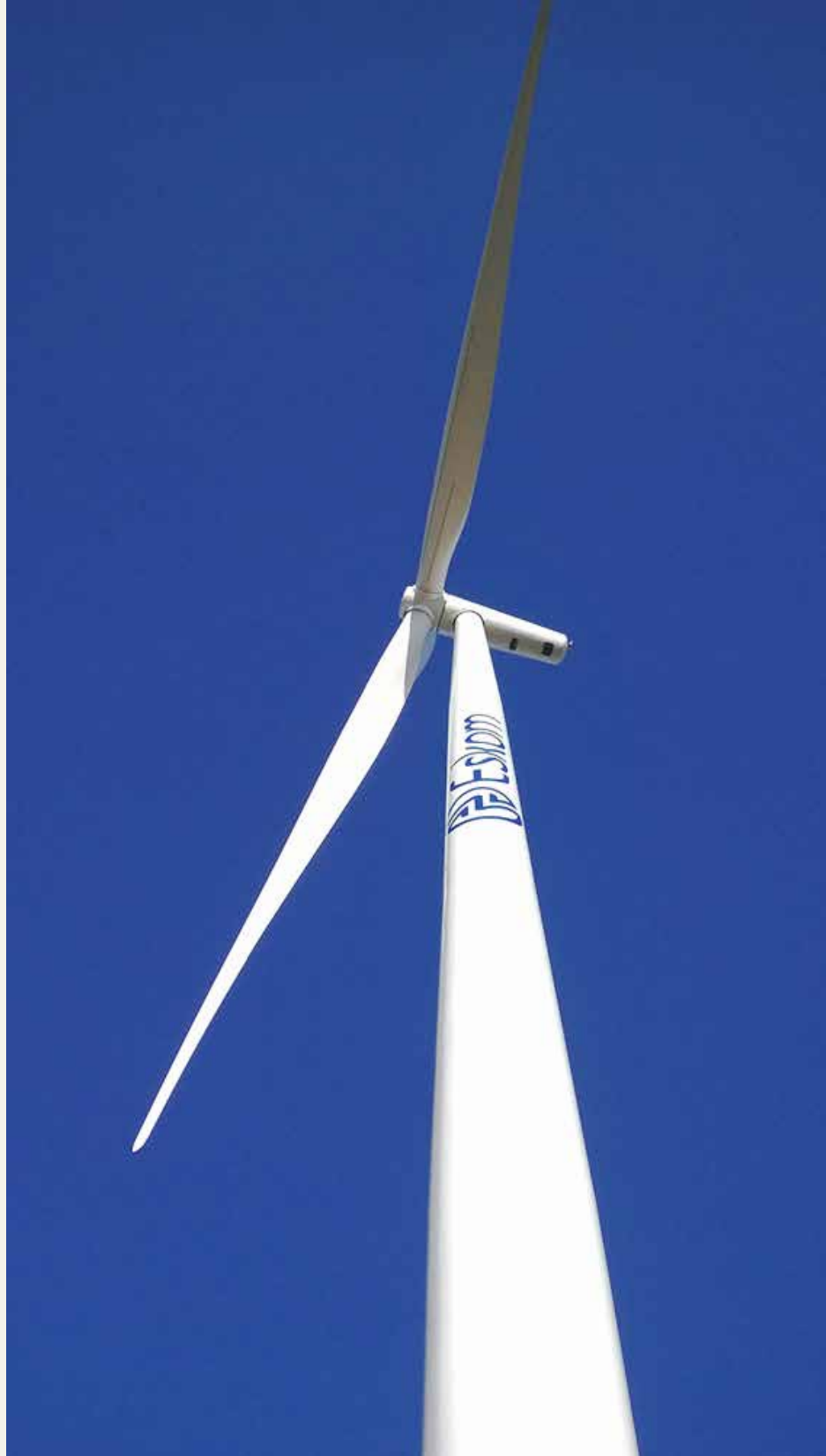
Figure 25: One of the 46 Siemens 2,3VS-108 turbines at Sere wind farm, rated at 2.3MW each. Eskom, South Africa (STERG 2014c).
