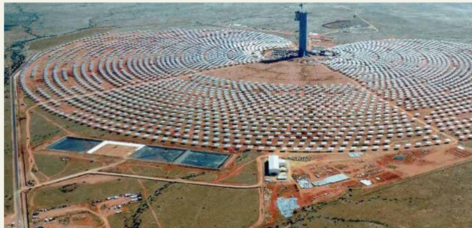
Figure 12: Khi Solar One: 50MW central receiver. Abengoa, South Africa (Abengoa 2014b).
