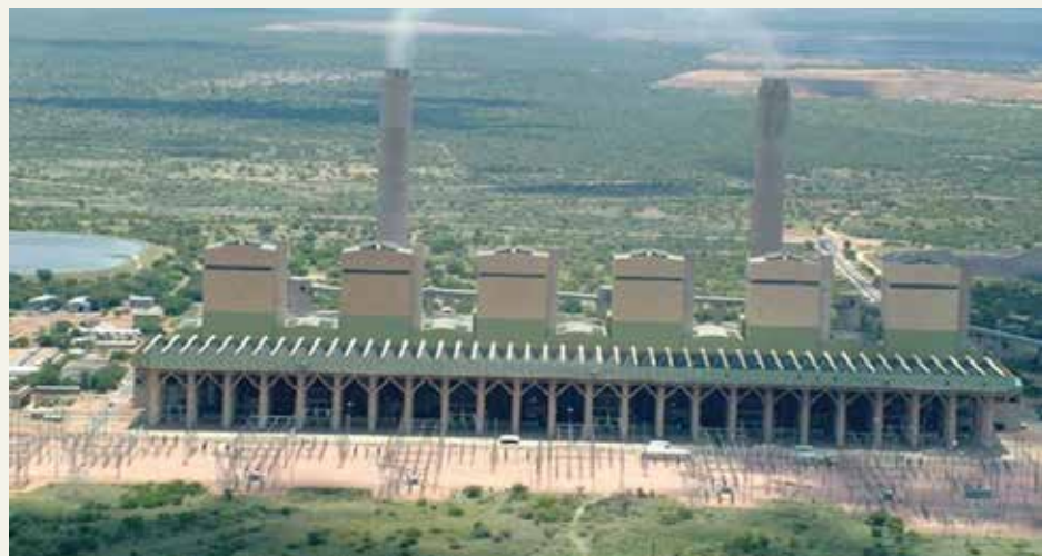
Figure 4: Matimba 3990 MW direct dry-cooling coal power plant. Eskom, South Africa (Eskom 2013).
