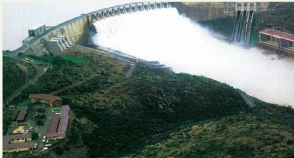
Figure 5: Gariep 360MW hydroelectric power plant. Eskom, South Africa. (Eskom n.d.a).
