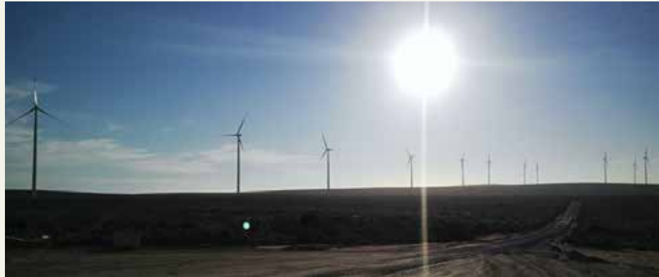
Figure 9: Sere 100MW wind power plant. Eskom, South Africa (STERG 2014b).
