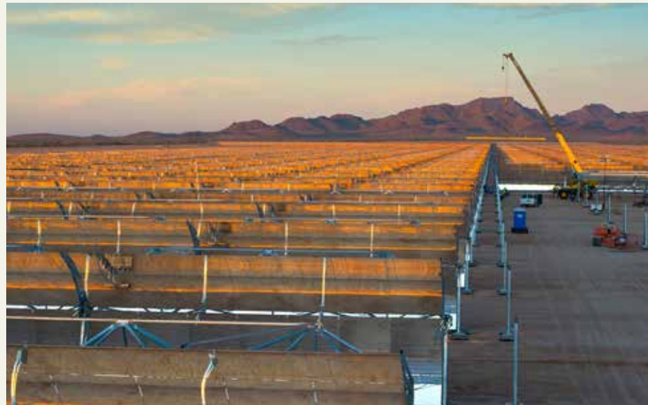
Figure 13: Solana 280MW parabolic trough power plant in Arizona, Abengoa, USA (NREL 2012).
