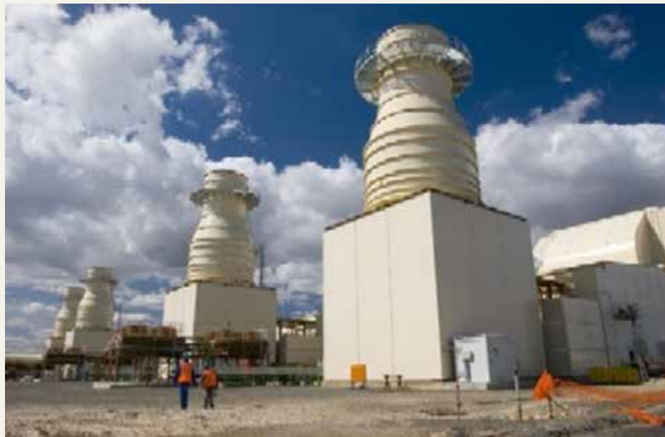
Figure 7: Ankerlig 1338MW open cycle gas turbine power plant. Eskom, South Africa (Eskom n.d.c).
