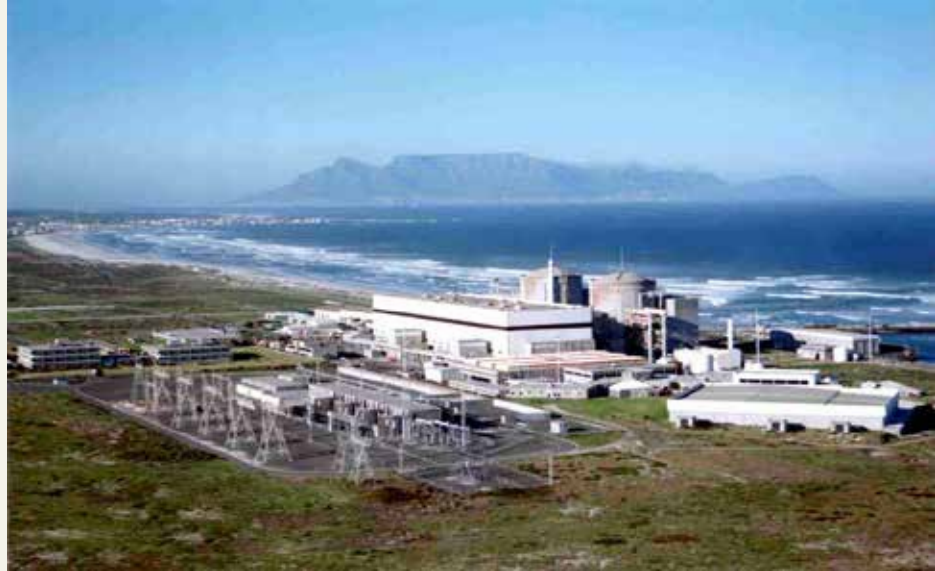
Figure 6: Koeberg 1800MW nuclear power station. Eskom, South Africa (Eskom n.d.b).
