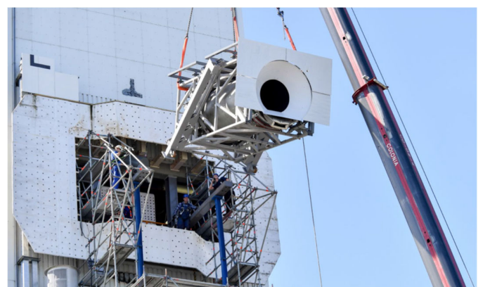
Fig. 9: The CentRec 1\text{ m}^2 prototype receiver during installation in Jülich [10]
