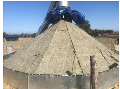
Fig. 11. Fitment of insulation
