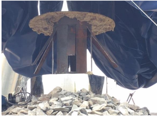
Fig. 8. Modification of hot air inlet pipe
