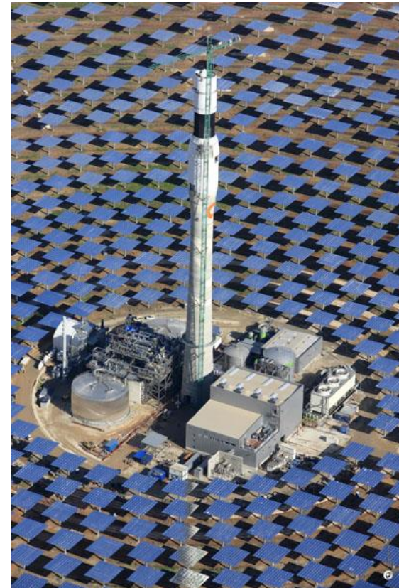
Figure: Solar Salt receiver and storage tanks of the Gemasolar plant
