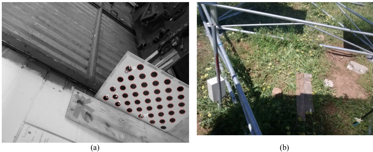
FIGURE 1. Sample Photo from back of Heliostat. a) In workshop with optical target. b) In the field observing the pod base
